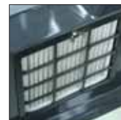
Internal air conditioner filter
